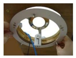
2. Position the retaining brackets to hold the mount on the ceiling.
